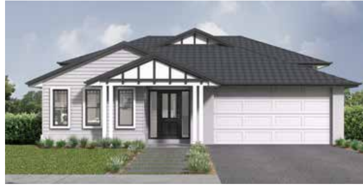
Hamptons Facade Roof Type Tiles Total m 2 /Sq 267.89/28.8
