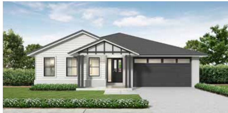
Hamptons Facade Roof Type Tiles Total m 2 /Sq 245.51/26.4
